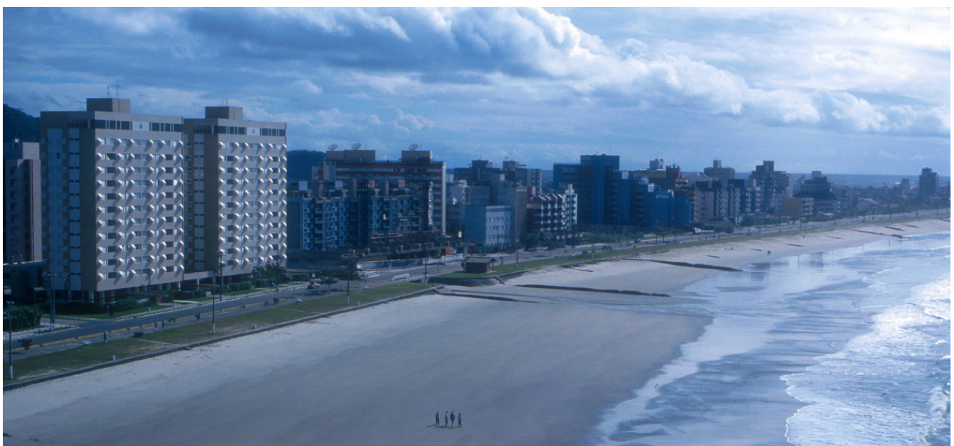
Figure 22. Gabion sea-walls, jetties and groins at Caiobá-Matinhos beach-arc in 1994 (see location in Figure 1).
