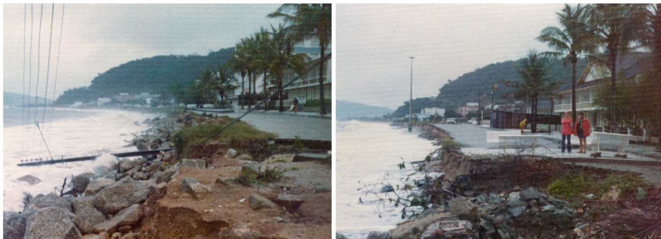
Figure 18. Two views of Beach erosion at Praia Mansa in 1976 (After Emopar, 1978; see location in Figure 1).
