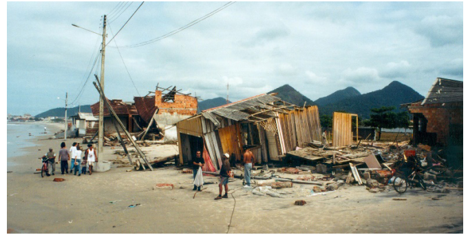
Figure 28. Damage caused by a high energy wave event associated with both spring tides and storm surge in Matinhos in May of 2001 (After Angulo et al. , 2006b; see location in Figure 1).
