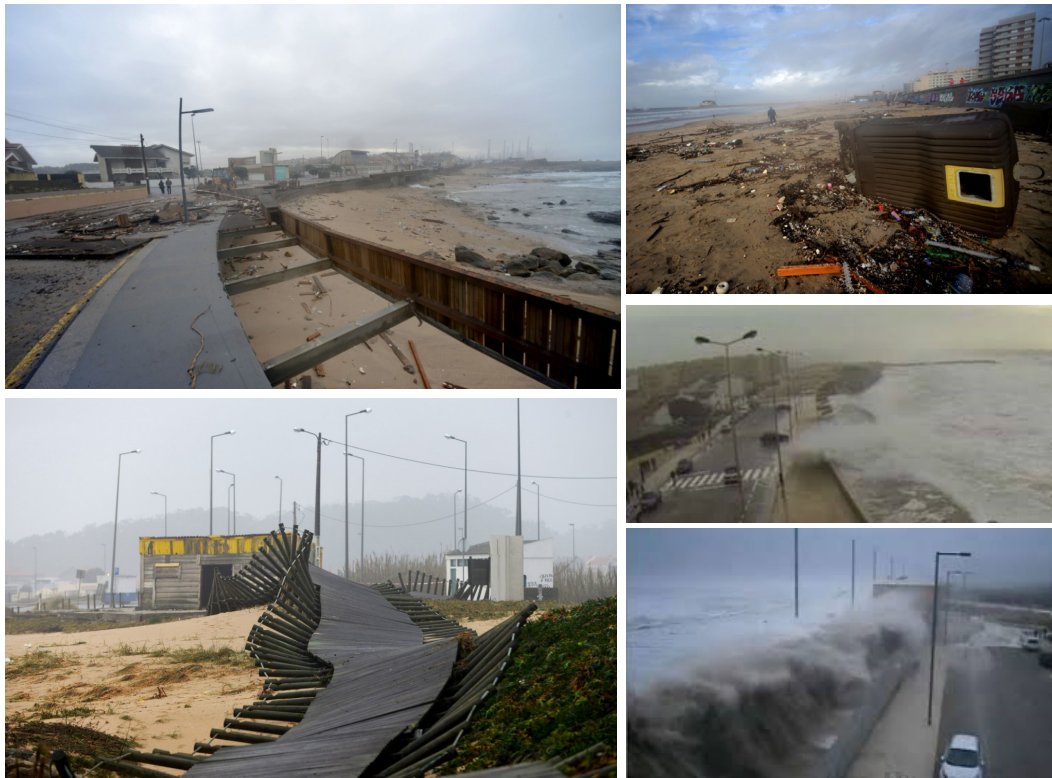
Figure 5. Damage in the NW coast of Portugal due to the storm of January 3-7, 2014. Examples from Matosinhos, Porto, Gaia and Furadouro (source: Público Newspaper).
